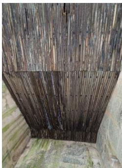
The ceiling is laminated (layered) with wood and metal. The layering and the shape of the ceiling is believed to have been to direct any ricocheted shells/fragments back into the butt to land safely in the sand.
